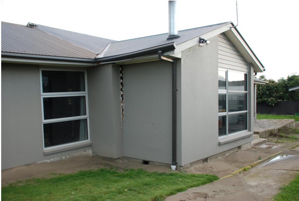
Figure 11 – A “tear” in the walls of a house caused by liquefaction-induced ground settlements. This happened when liquefaction caused the house to settle unevenly. Houses in this area will be abandoned. Repair or rebuilding was not feasible.
