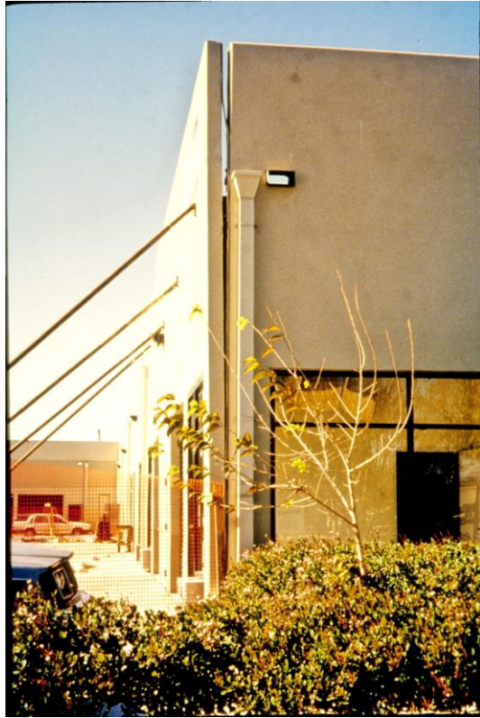
Figure 12 – An example of wall separation from the roof of a building. When this happens, the walls can fall over, the roof can collapse locally, or both can happen.
