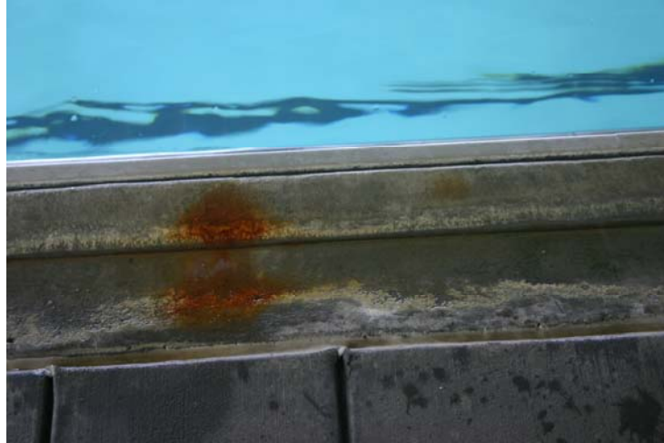
Existing Stainless Steel Gutter
